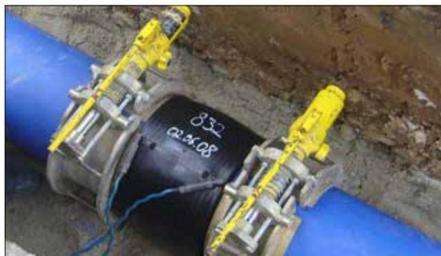
6.81 Re-rounding clamps for EF joints (source: +GF+)
