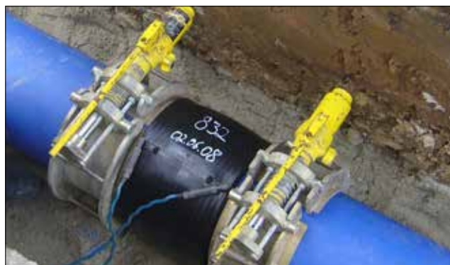
6.81 Re-rounding clamps for EF joints (source: +GF+)
