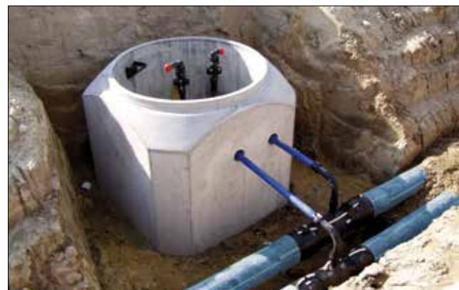
6.80 Tapping fittings for manhole connection
